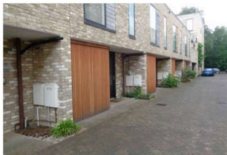
Utility meters mounted on oblique facing wall with provision of landscape planter for additional screening.
