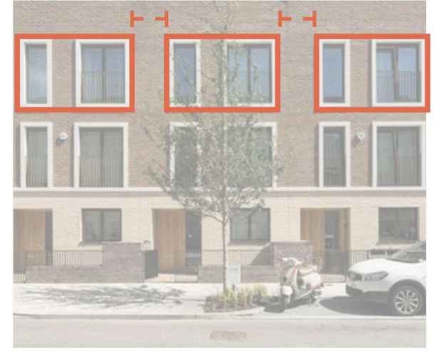
Precedent: Coordinated windows along the building's facade. Chobham Manor.
