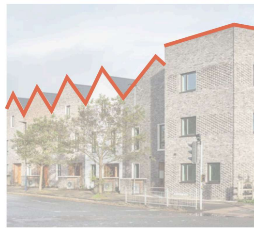
Precedent: Flat roof building defines the corner plot. Marmalade Lane.
