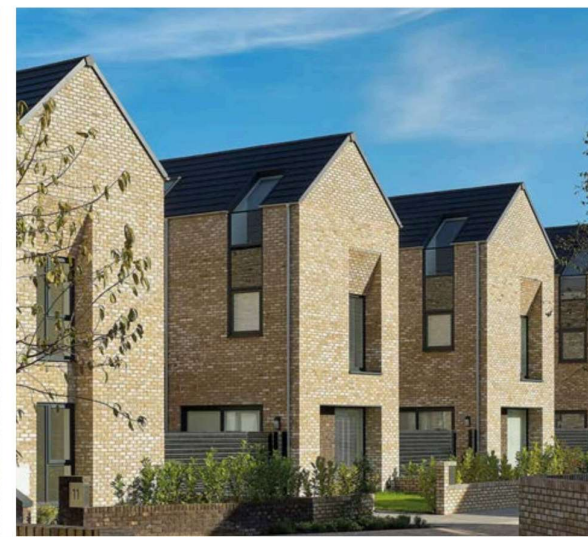
Precedent: Buff brick with contrasting grey roof tiles. The Gables, Crosby.
