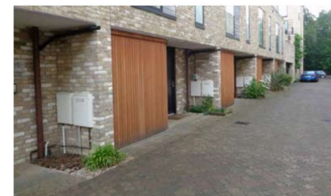
Utility meters mounted on oblique facing wall with provision of landscape planter for additional screening
