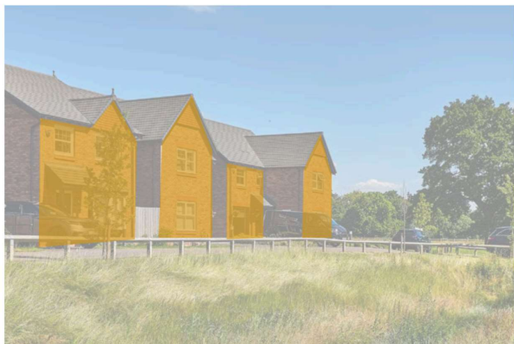
Precedent: Buildings facing adjacent open space and woodlands. Heathfields Farm, Wilmslow.
